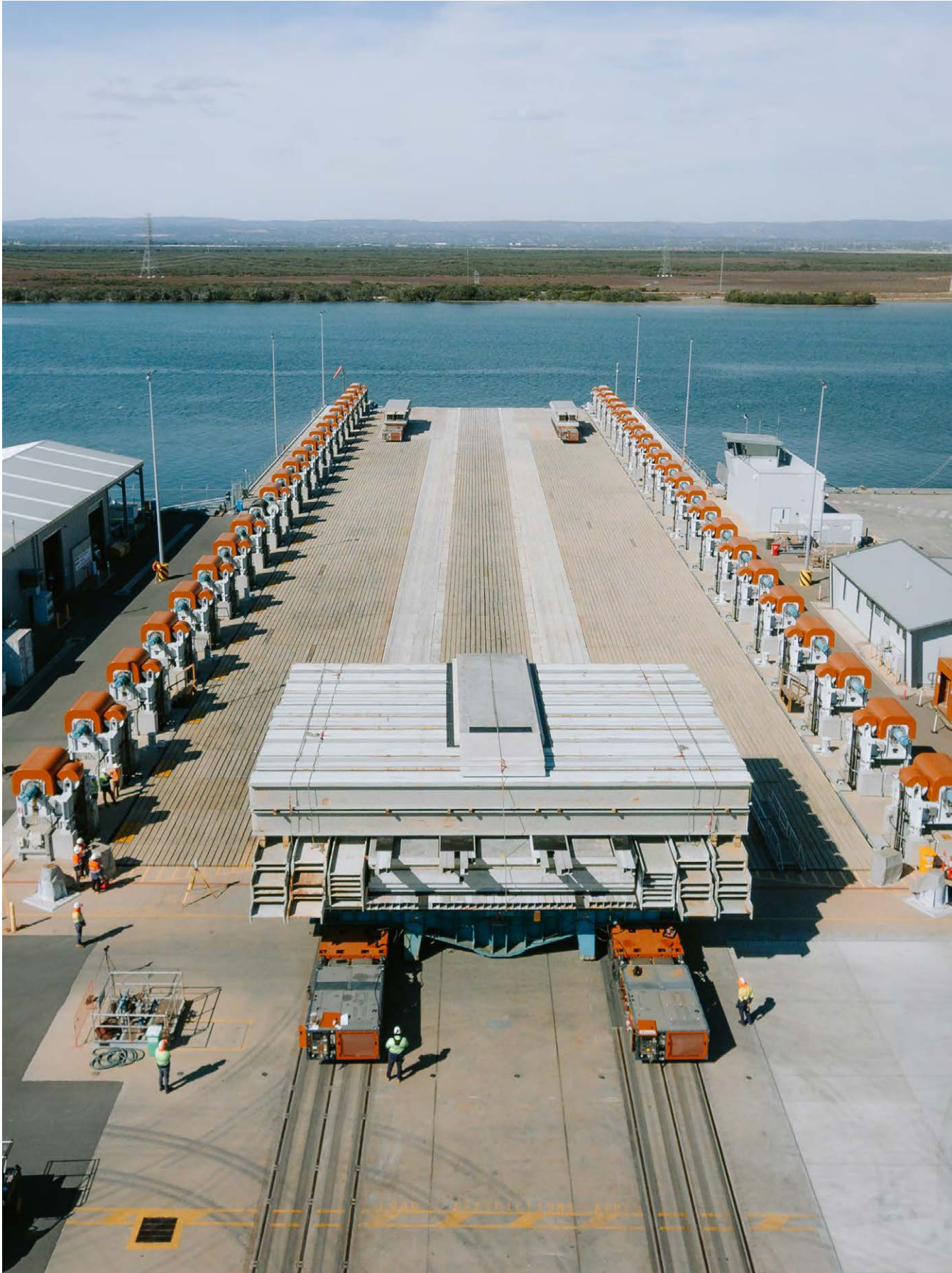
Shiplift load testing
