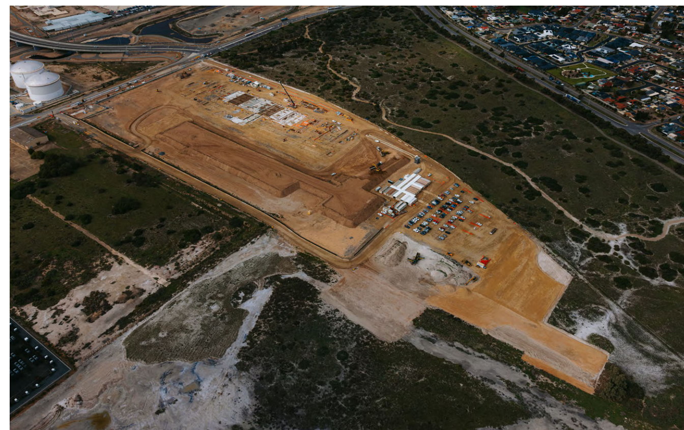
Aerial view of the STAC construction
