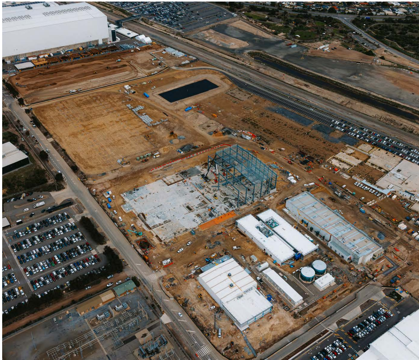
Aerial view of construction underway in Area 1
