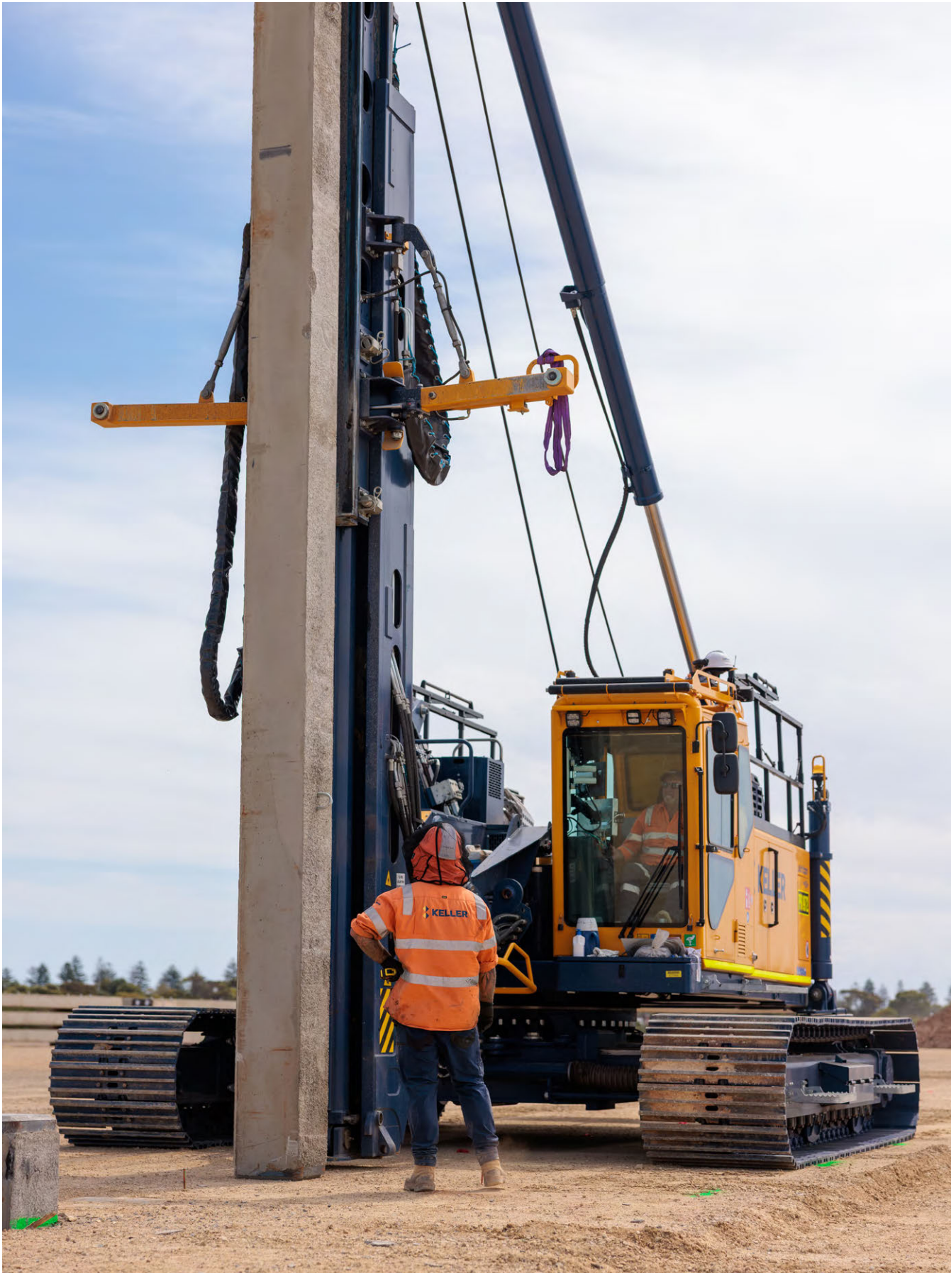
Pile being driven into the ground at the STAC site
