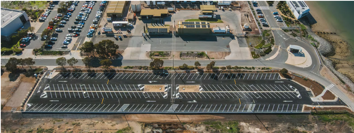
Aerial view of newly constructed P6 carpark for BAESMA
