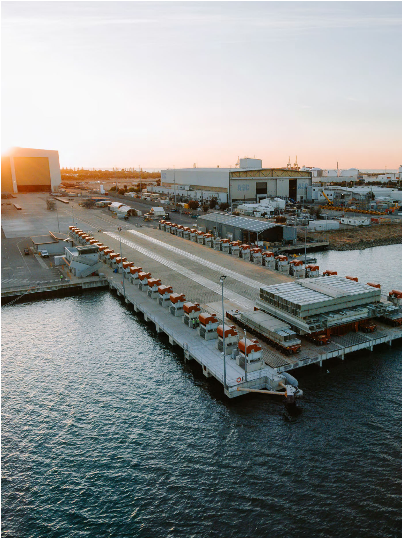
Shiplift load testing
