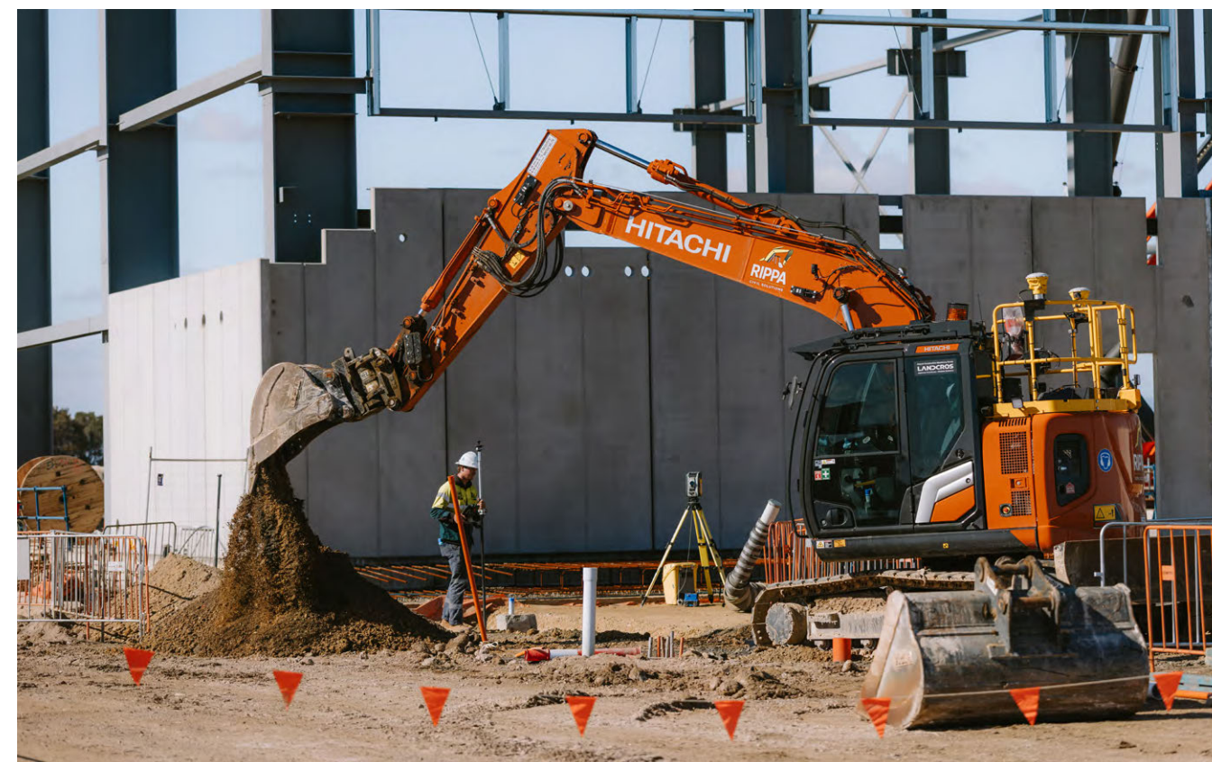
Area 1 construction on Building N110 underway
