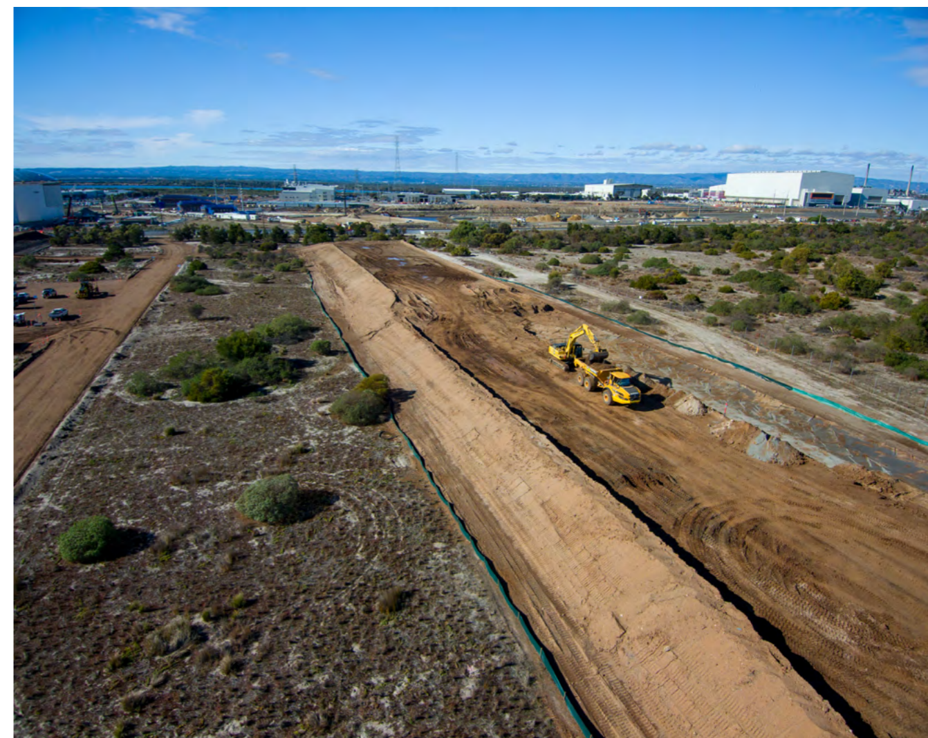
STAC site preparation works
