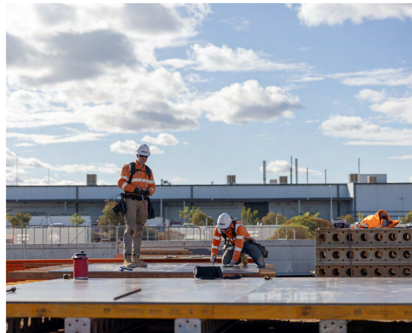
Link Road under construction
