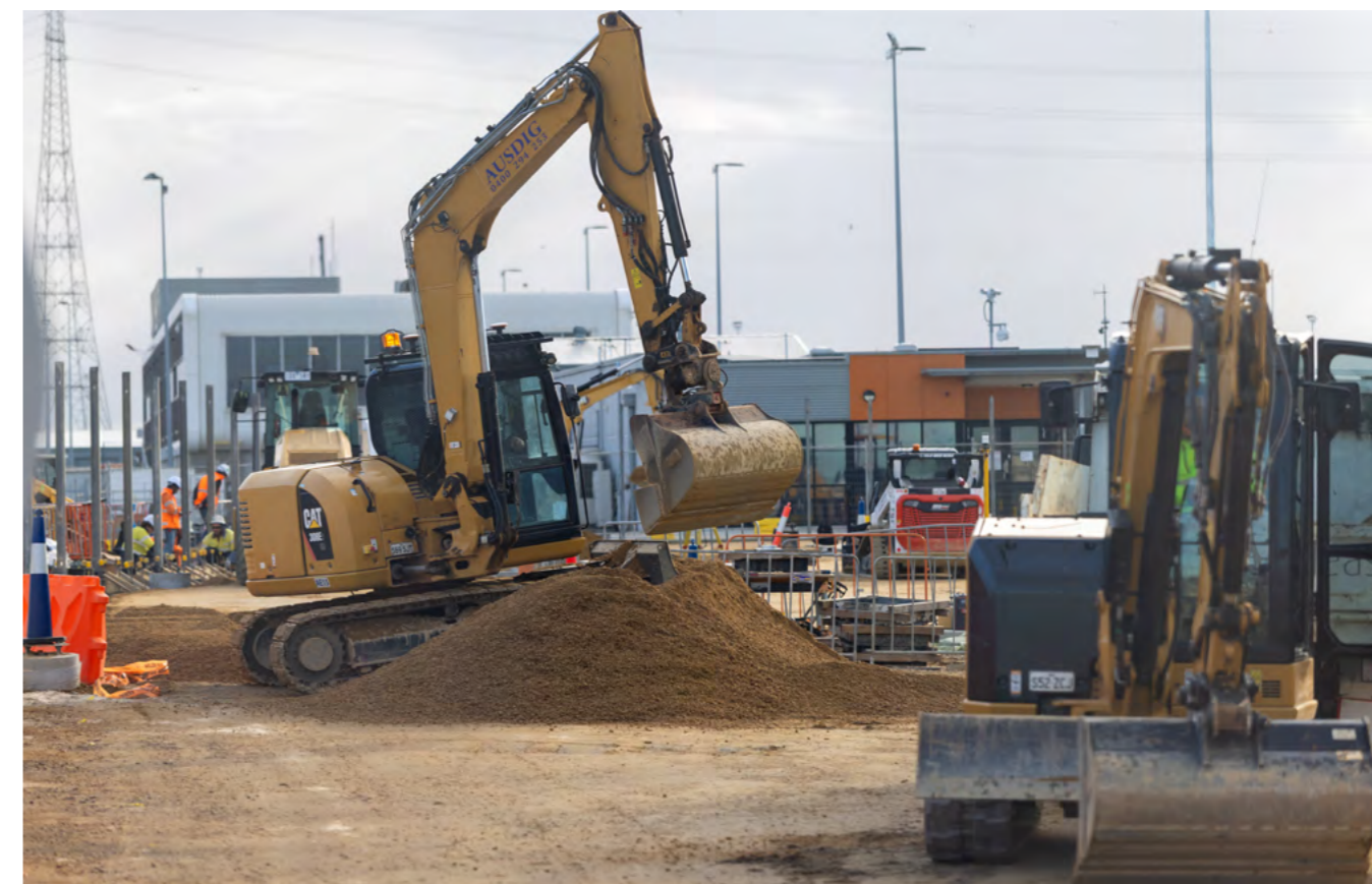
Eastern entry works under construction
