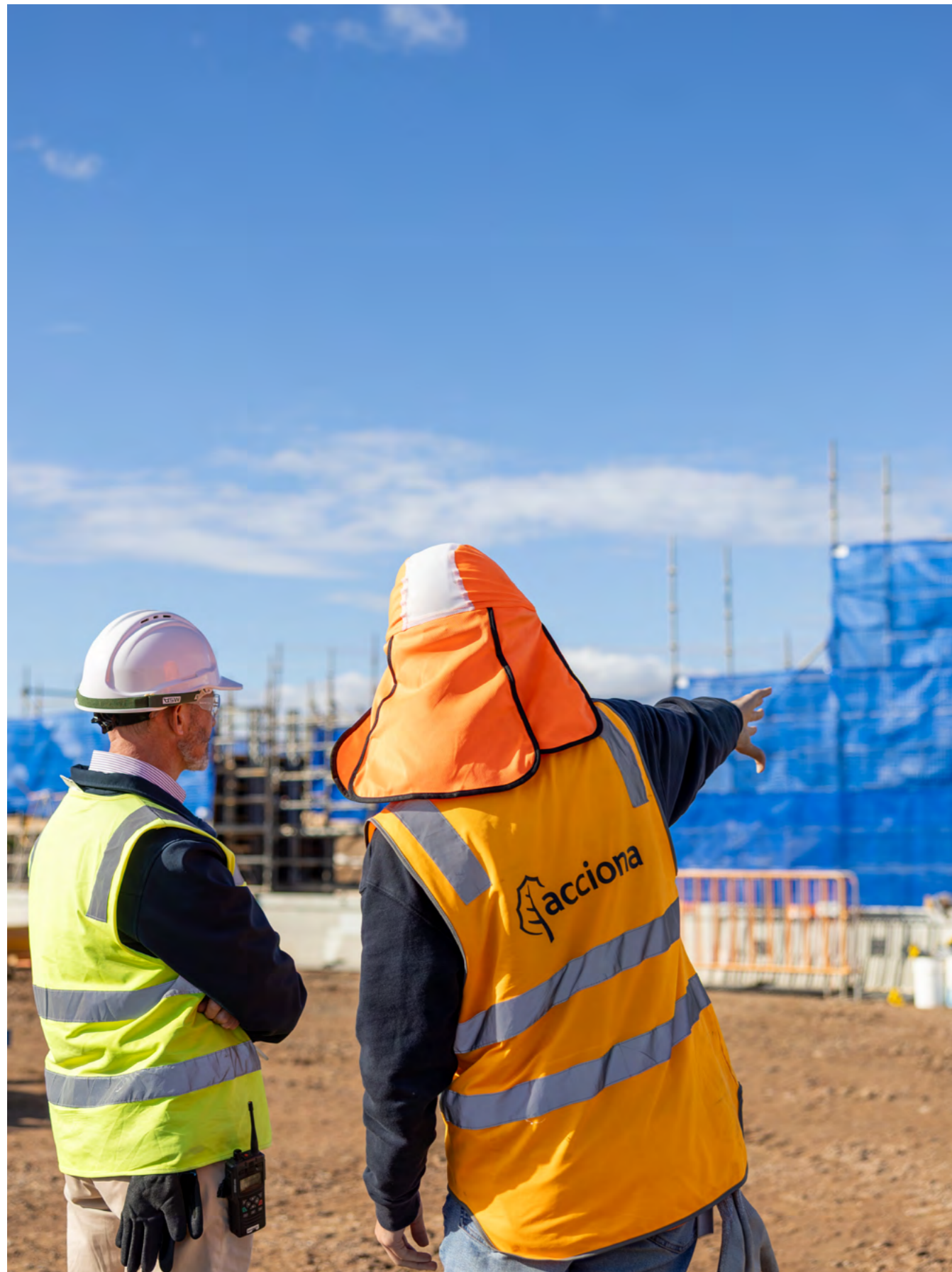
Link Road construction
