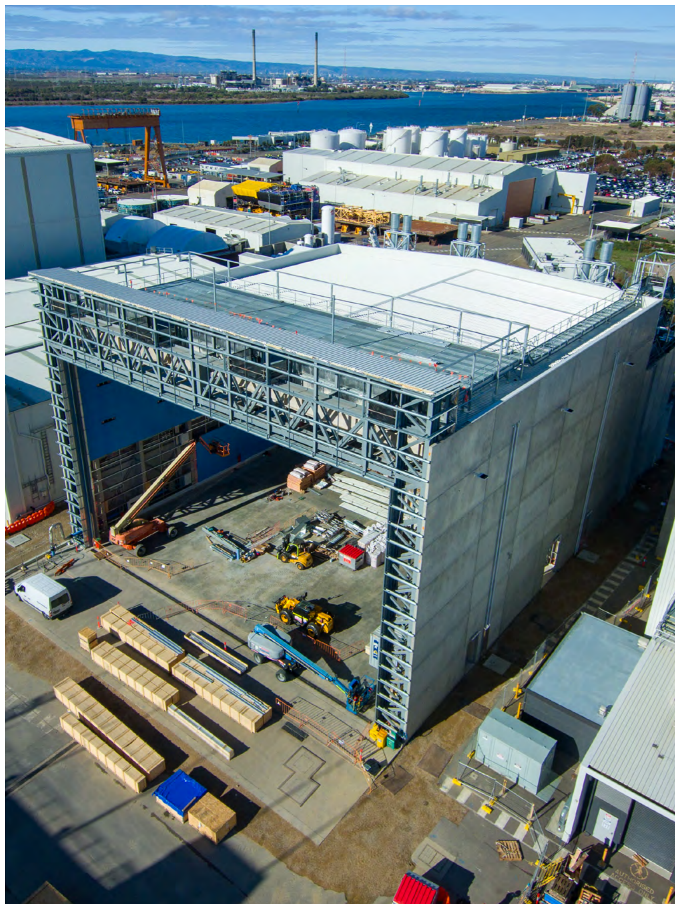
Blast and paint facility (Building 18A) under construction
