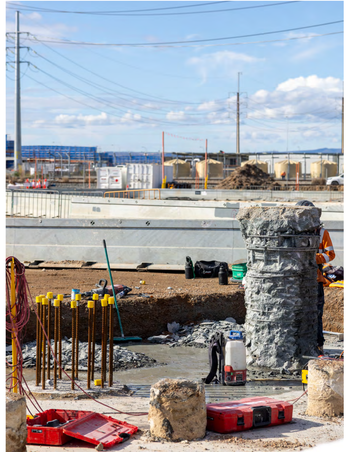
Link Road under construction
