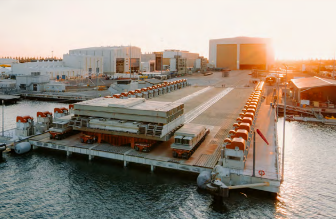
Load testing the newly upgraded CUF shiplift
