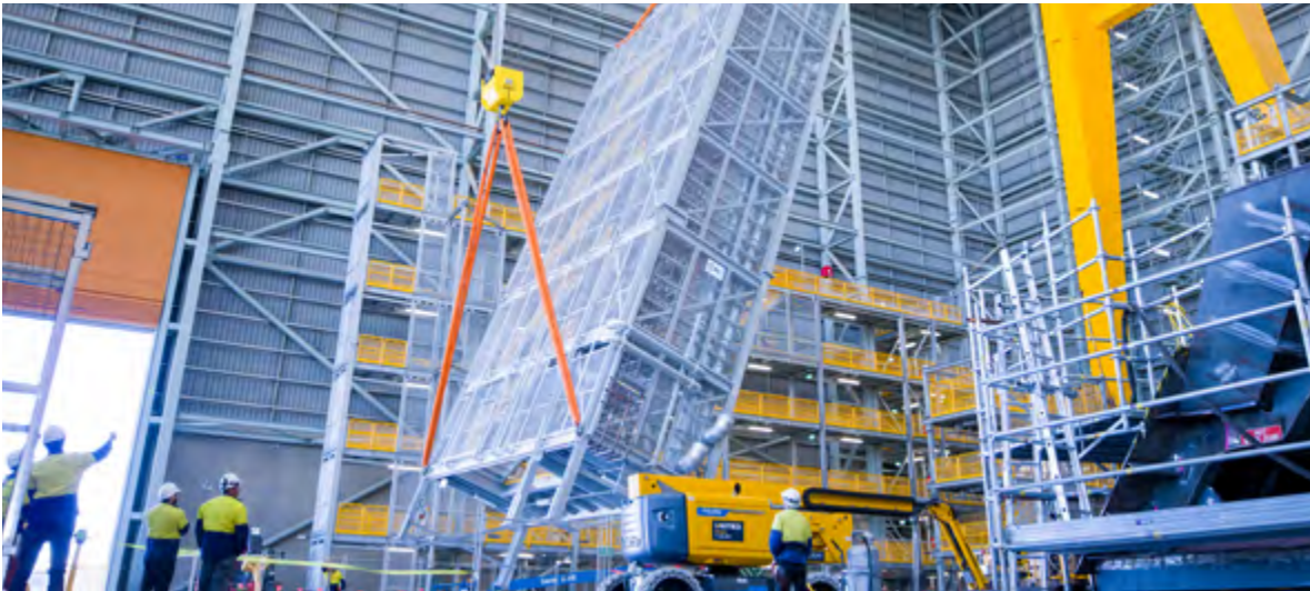
Support tower being moved into place within Building 22
