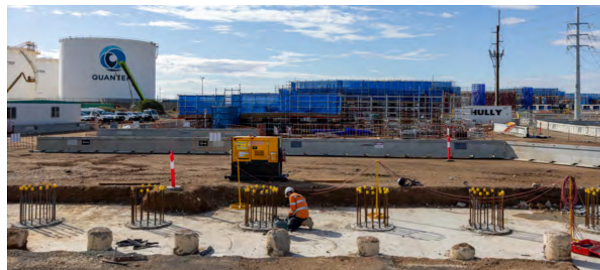
Link Road under construction
