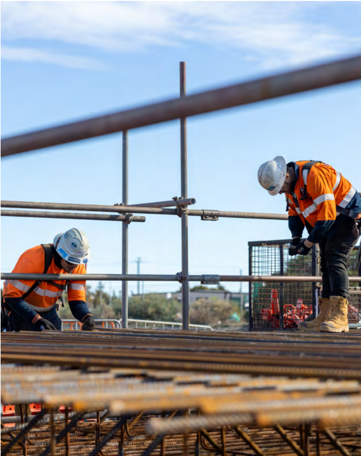
Link Road bridge under construction
