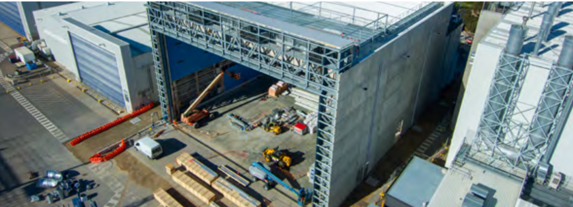
Blast and paint facility under construction
