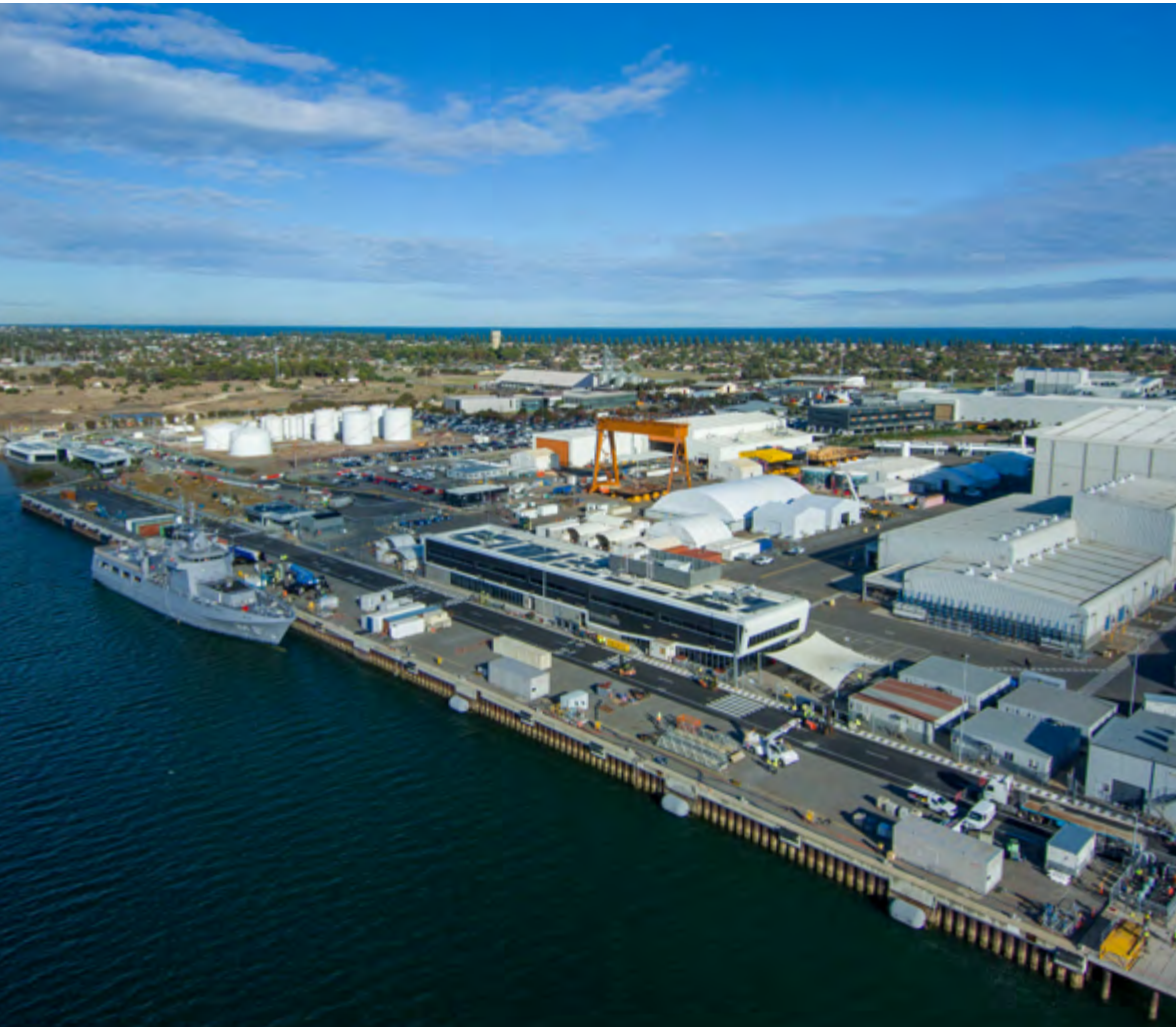
Aerial view of completed wharf extension at ONS-5
