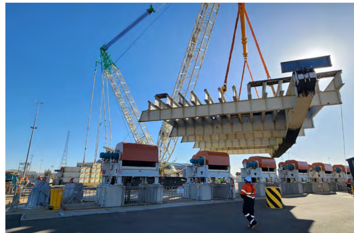
Shiplift platform lift
