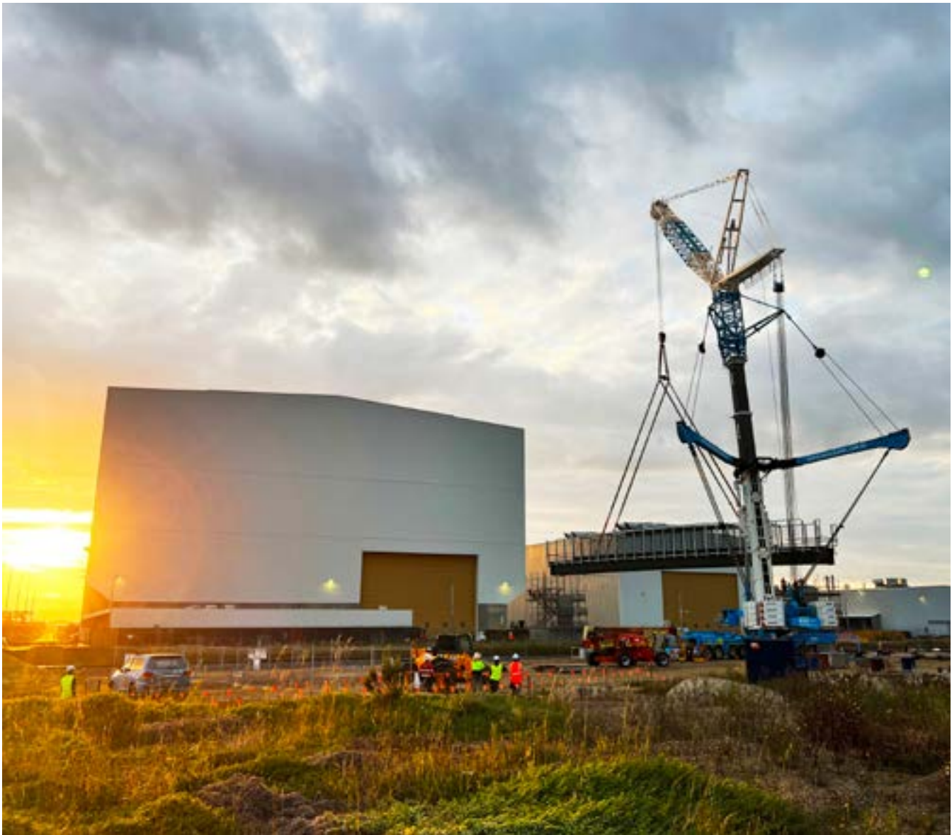
ONS-S pedestrian bridge lift over rail corridor
