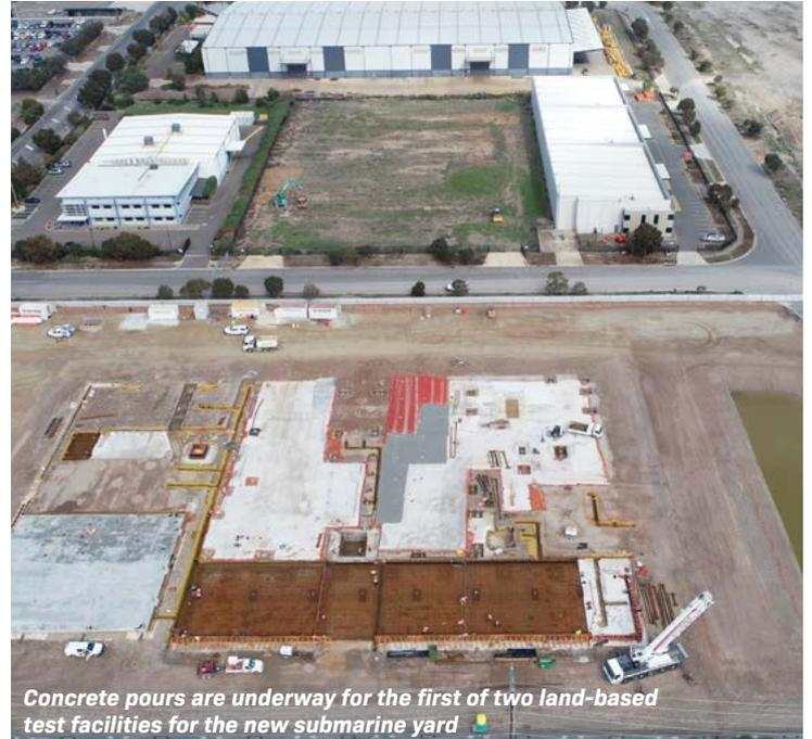
Concrete pours are underway for the first of two land-based test facilities for the new submarine yard
